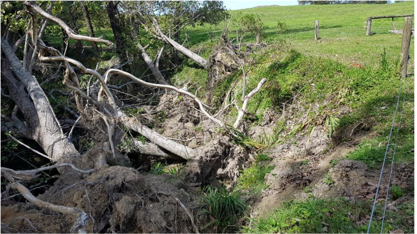
Eroding bend with toppled trees.
