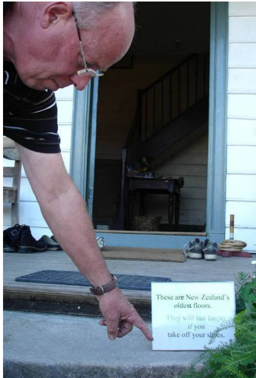
Figure 7: Flood level at Kemp House.
