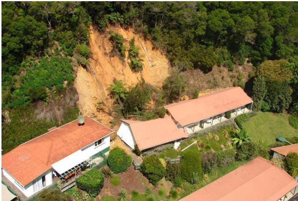
Figure 15: Landslide damage to the back of Haruru Falls Resort. (Photo FNDC)
