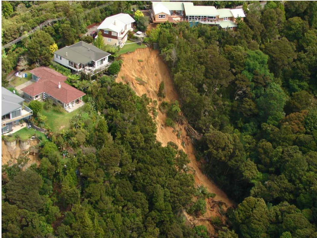
Figure 4: Slope failure at Opuia on 29 March, 2007 (FNDC Photo).
