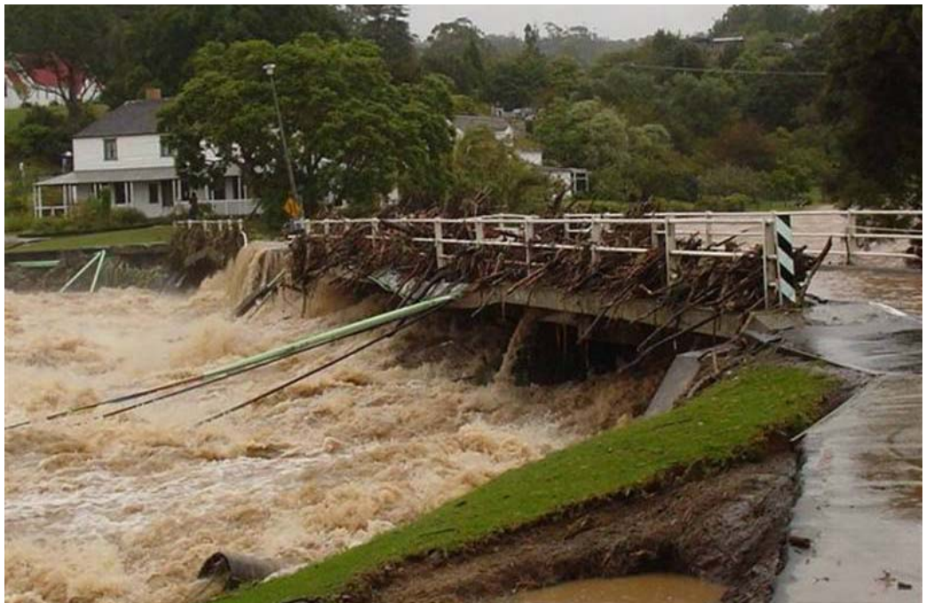
Figure 9: Flood debris on the Kerikeri Basin bridge, Kemp House in background. Photo: FNDC.
