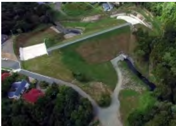
Whangārei's Hopua te Nihotetea detention dam.
